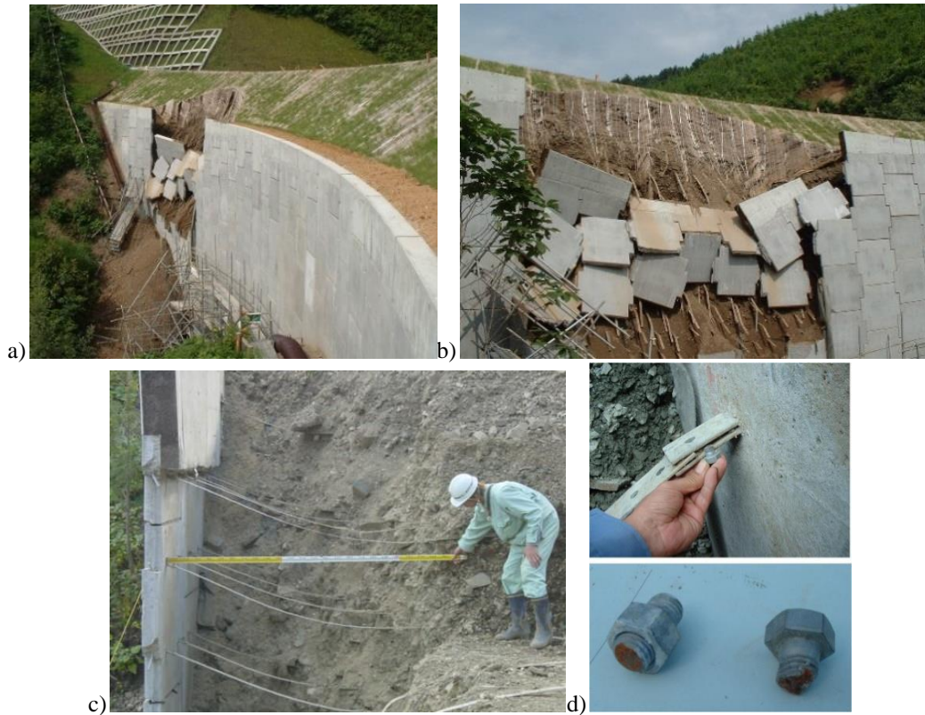
Figure 3-3. Collapse of a Terre Armée RW for an approach road to an irrigation dam in Aomori Prefecture, August 2001 (constructed February 2001): a) overview; b) front view; c) excavated cross-section; and d) typical sheared-off connection.
