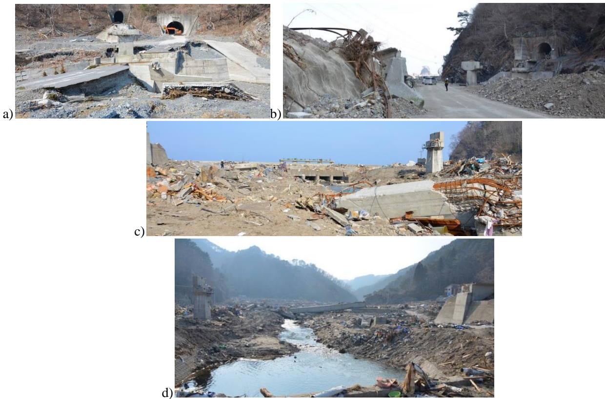
Figure 6-5. Three bridges for Sanriku railway washed away by tsunami during the 2011 Great East Japan Earthquake: a) Haipe; b) Koikorobe; and c) (from inland) & d) (from seaside) Matsumae-gawa adjacent to Shimanokoshi Station: at the end of March 2011; see Fig. 3-16d for the locations of these sites (by the courtesy of Japan Railway Construction, Transport and Technology Agency).
