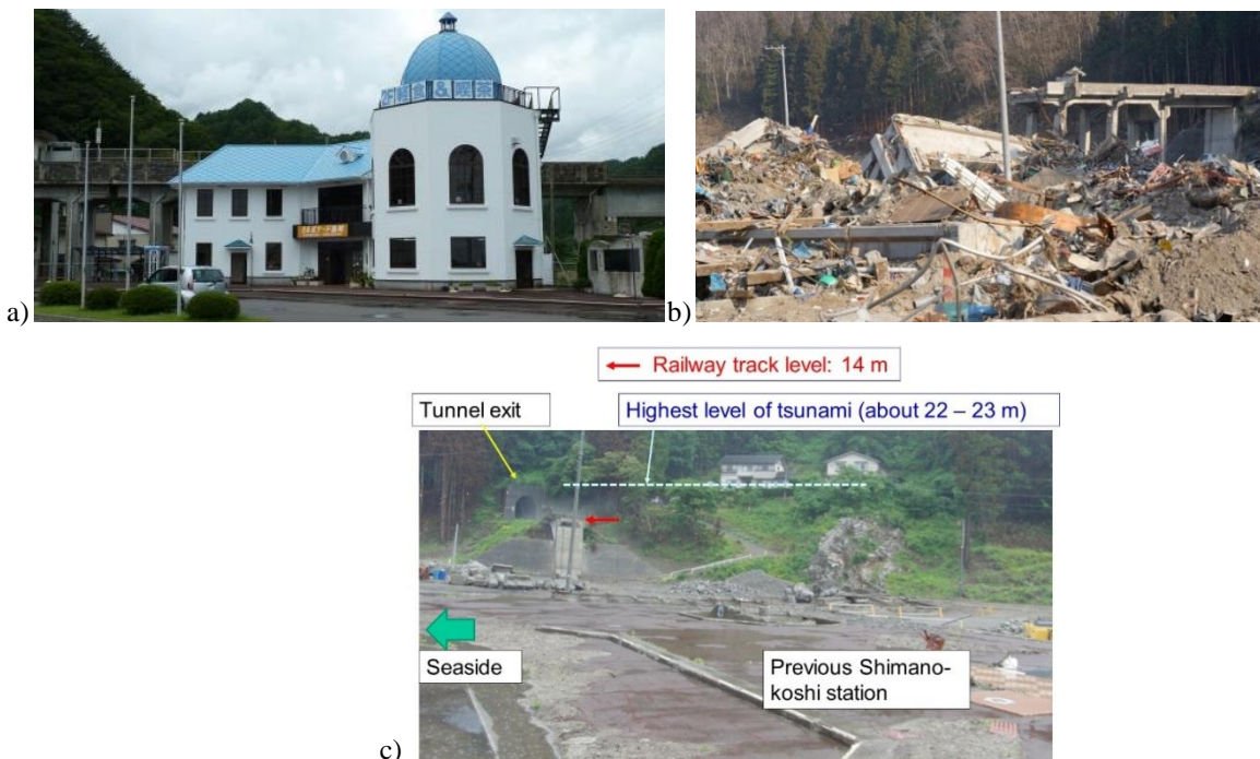
Figure 6-11. Shimano-koshi Station area, Sanriku Railway (see Fig. 3-16d for the location) seen: a) from the seaside before the earthquake; b) immediately after the earthquake seen from the inland, 30 March 2011; and c) from the seaside, 14 July 2013.
