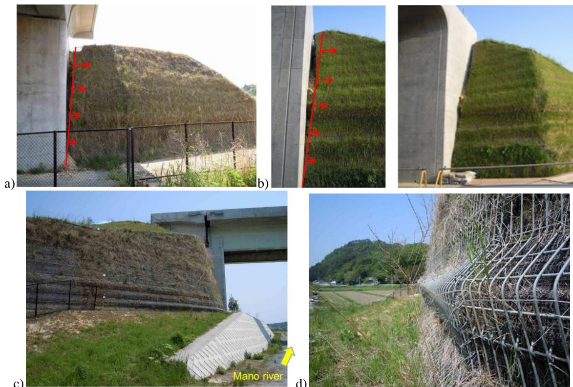
Figure 2-10. Performance of GRS RW with wire mesh facing at: a) restorability limit state; b) serviceability limit state; and; c) overall picture and d) zoom-up of buckling deformation of metal mesh facing of GRS RW for a wing of a bridge abutment of an expressway (under construction) in Minami-Soma, Fukushima Prefecture (Kuwano et al., 2014).
