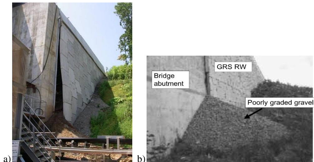
Figure 2-8. Large deformation of discrete panel facing, Iwate Prefecture during the 2008 Iwate-Miyagi Nairiku Earthquake; a) Terre Armée RW, Isawa, Iwate Prefecture; and b) GRS RW (Wang et al. 2011).
