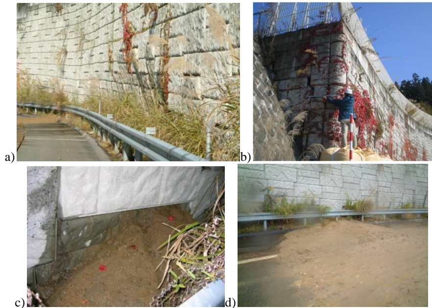
Figure 3-5. Terre Armée wall (5 – 9 m-high & 100 m-long, constructed 1997) along a ramp at Horinouchi interchange, Kantetsu expressway, damaged during the 2004 Niigata-ken Chutsu Earthquake (Kitamura et al., 2006): a) & b) views of the wall; and c) opening between panels from which a large amount of liquefied sand spouted; and d) sedimentation of sand in front of the wall.
